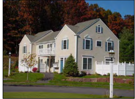
Avon, CT – Old Farms Crossing, 45-units of rental housing Source: Partnership for Strong Communities
